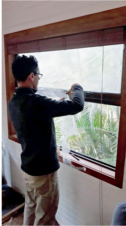
Left: Draught seals on a sliding window—a foam product from Raven and some self-adjusting perimeter seal, known as “EMV”. Right: insulating a window with bubblewrap, AKA bubbleglazing.
