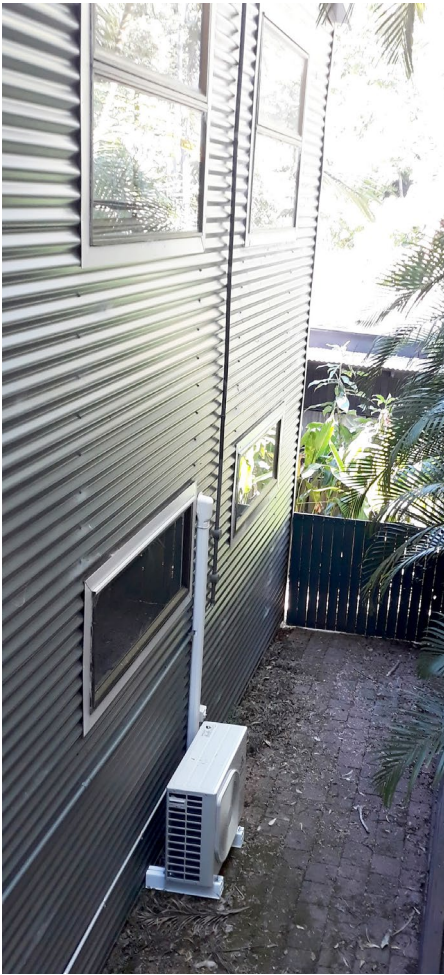
Wall insulation was added when the walls were reclad.
