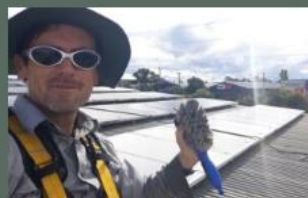
Solar Panel Cleaning
